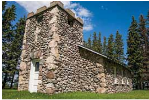
St. Paul's Anglican Church; (opposite) chalet at Moose Mountain Provincial Park.
